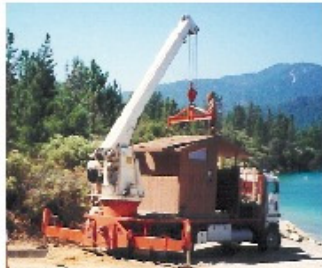
Installation by safe professional crews.
